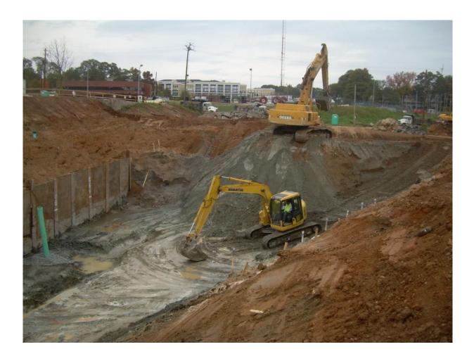
During the course of the project, lead-impacted soils were discovered within the footprint of the planned Site construction activities. Our professionals managed -- without incident and on deadline -- the excavation, transport, and proper disposal of approximately 35,000 tons of lead-impacted soil, from both on-Site and off-Site. These activities and their safety programs were reviewed by the Georgia Environmental Protection Division and subsequently issued regulatory closure.
