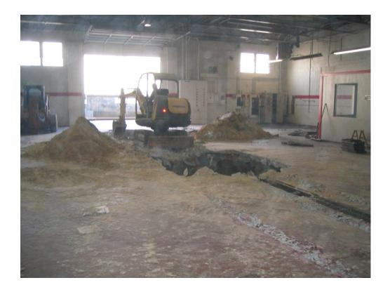
During the course of corrective action, several hundred feet of floor drains and sumps throughout the Site's facilities were removed and restored. All hazardous and non-hazardous wastes leaving the Site were characterized, profiled, and properly disposed into the appropriate landfills.
