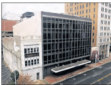
FORMER ALAGASCO, JR. LEAGUE, TOBY'S, BUILDINGS 1914-1926 First Ave. North $2 million
